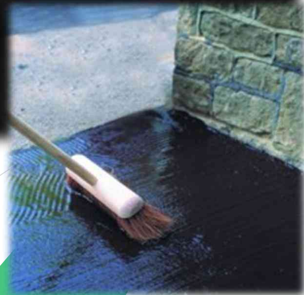
Bitumen Emulsion Application for Water Proofing
